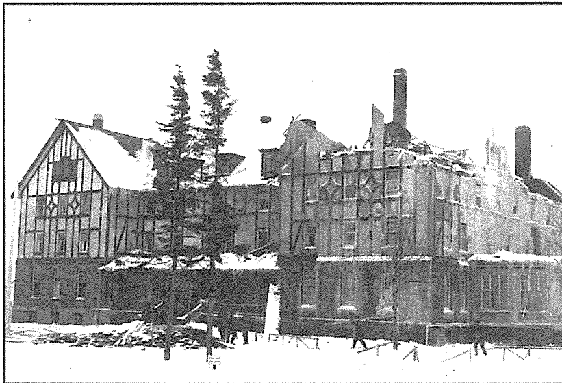
The Glynmill Inn after the fire in 1929
